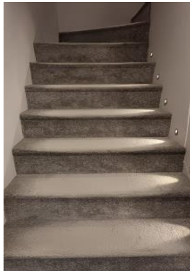
Fig. 4: Illuminated Grey Staircase Source: Photograph by Author
