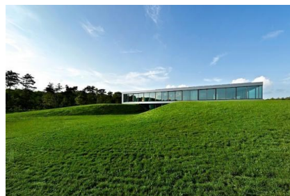
Fig. 2: Bridge House in Achterhoek, Netherlands
