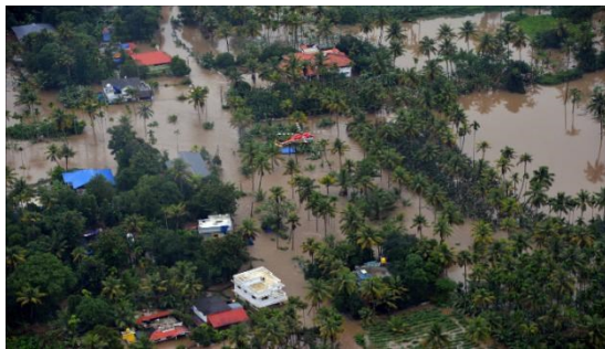
Fig. 14: Damage during Kerala floods, 2018 Source: Kerala Disaster Management
