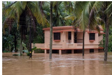
Fig. 15: Damage during Kerala floods, 2018 Source: Kerala Disaster Management
