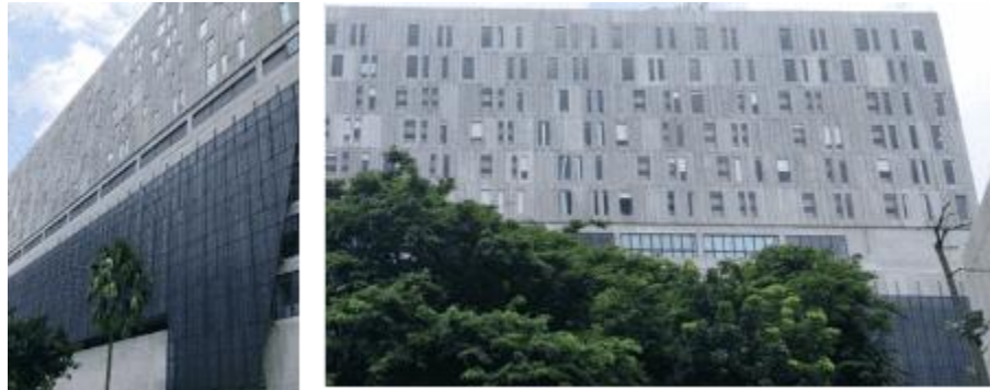
Fig. 5: The Building Facade of the Ali Sadikin Building Source: Author, 2023
