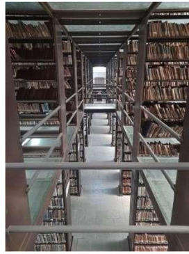
Fig. 8.2: Photograph showing the 1.2-meter-wide passage and 2-inch-thick Belgium glass measuring 90 cm x 75 cm.
