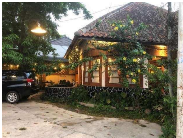
Fig 12: Documentation of the Building Facade 2
