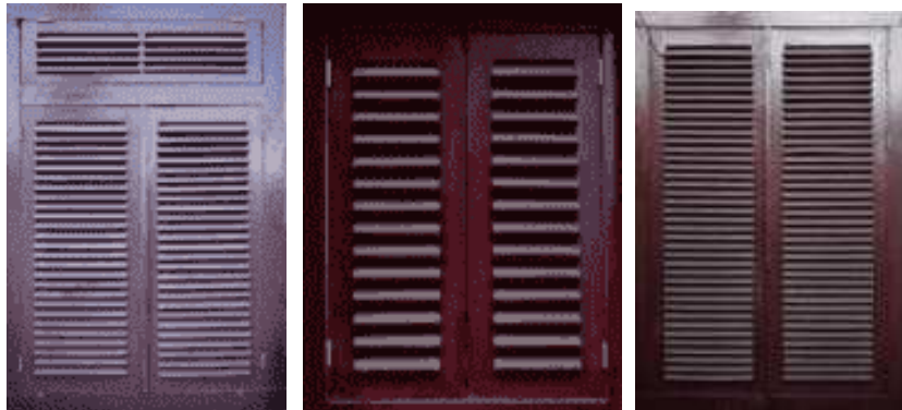
Fig 6: Indische Window and Fascade Source: Purnomo et al., 2017
