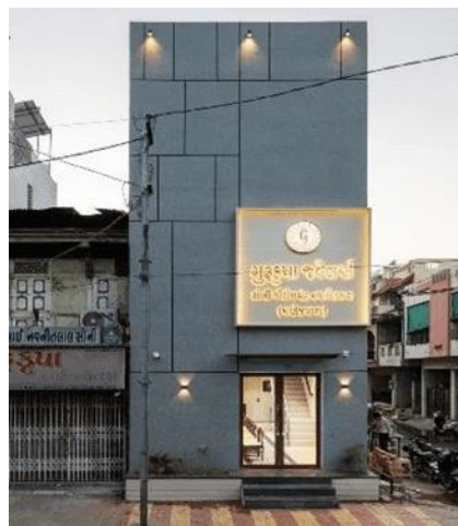
Fig. 14: Showroom Front Facade Source: Author
